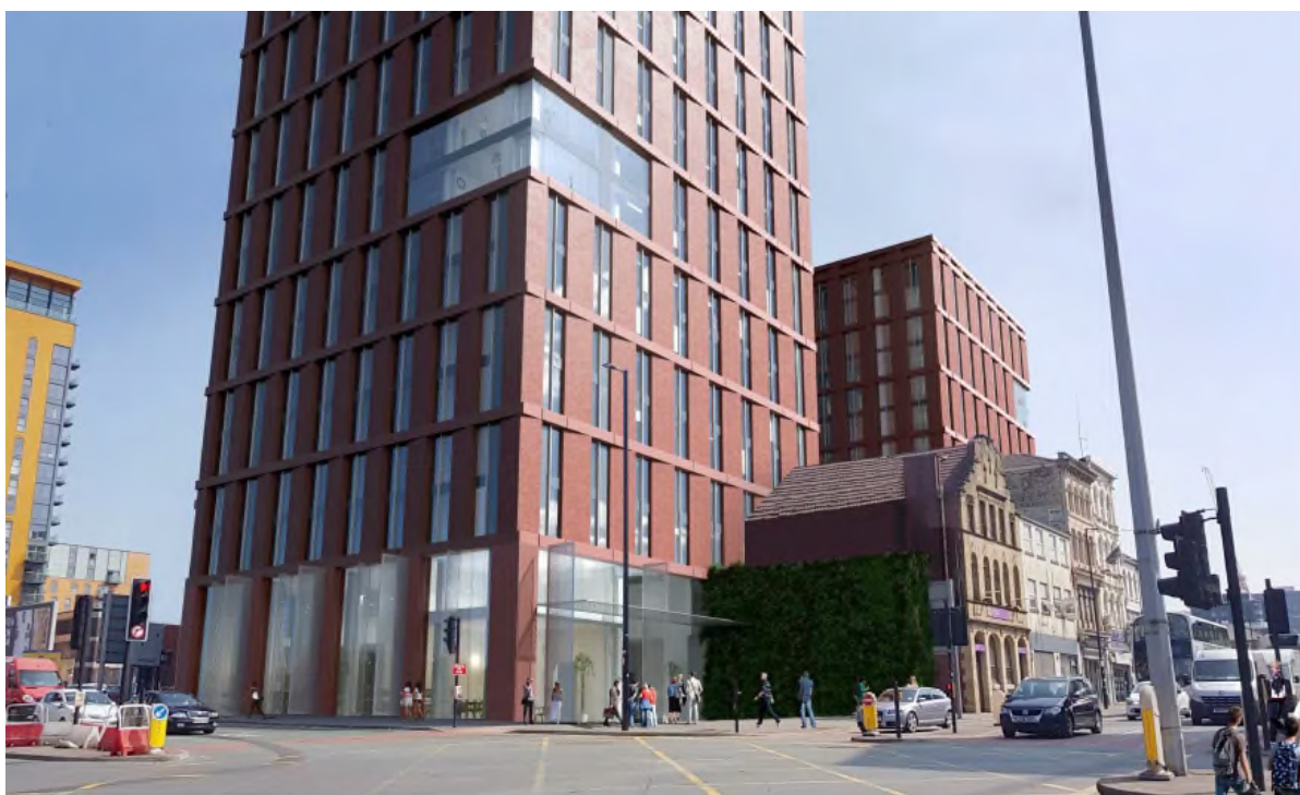
Main entrance to the western tower on the corner of Swan Street and Rochdale Road
