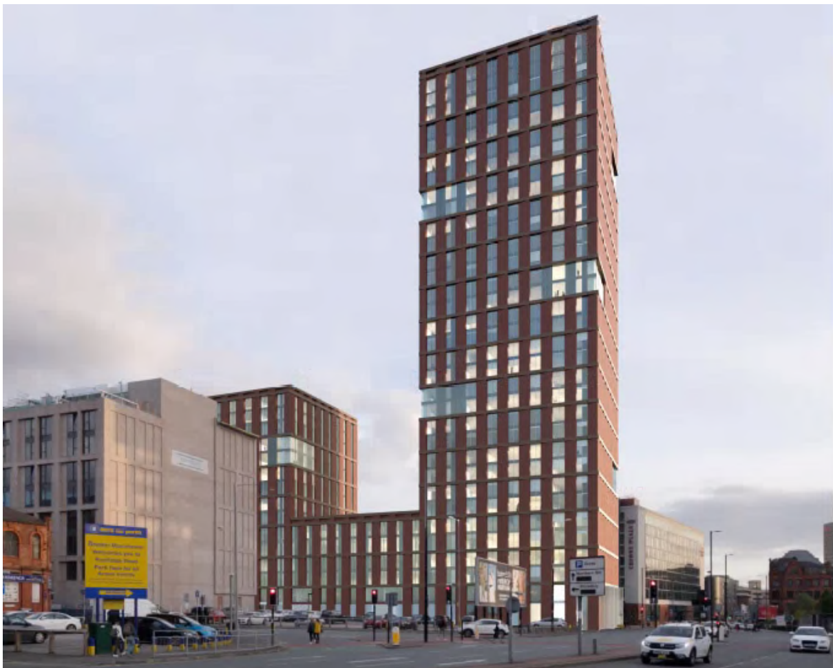
View of the building looking from Rochdale Road looking towards Shudehill (Marriott hotel to the left)
